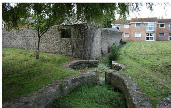
Figure 118: Remains of former flax barton at Allington Farm.
