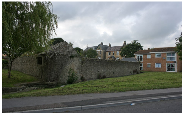
Figure 120: Former Allington Farm wall with Allington Farmhouse and Allington Vicarage in background.
