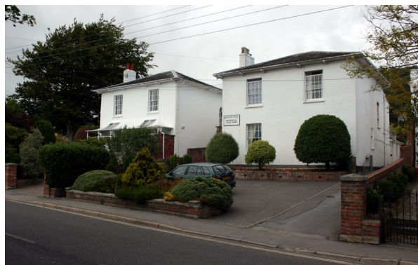
Figure 97: Late Regency/Early Victorian villas at 50 and 52 West Allington.
