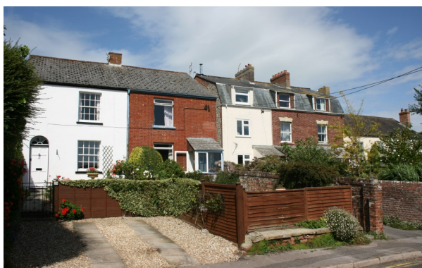
Figure 82: Nos. 16-29 Bedford Place.
