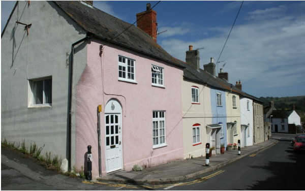
Figure 81: Nos. 2-10 Bedford Place.
