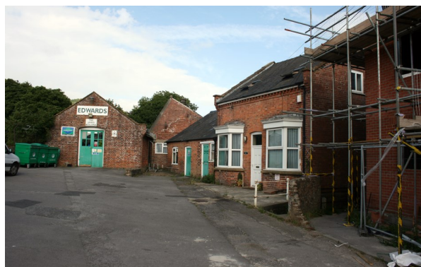
Figure 64: Edwards net factory, North Mills Road.
