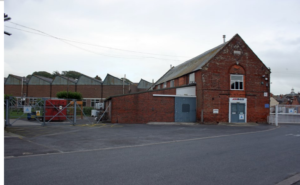
Figure 66: Industrial buildings at Court Mills.
