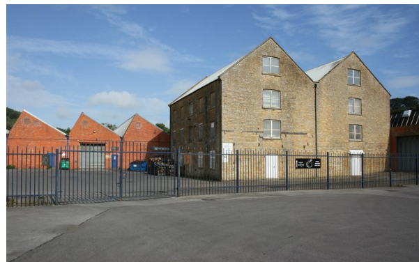
Figure 67: Warehouse and north-light sheds at North Mills.
