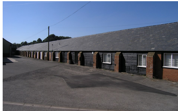
Figure 68: Covered Ropewalk, North Mills.
