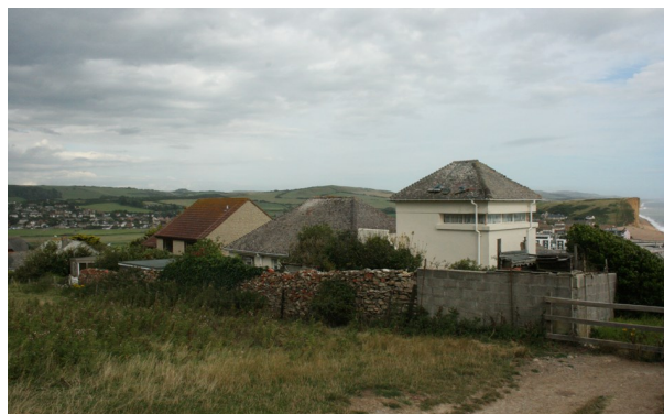
Figure 204: Former Battery Observation Post of WW2 coastal battery, West Cliff.
