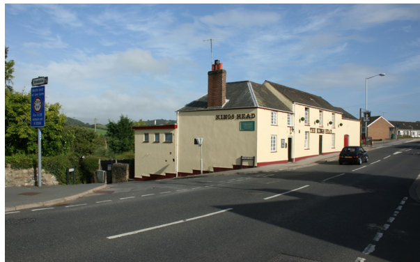
Figure 150: Kings Head Public House, St Andrews Road, Bradpole.
