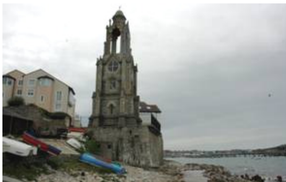
Figure 80: Wellington Monument with pillbox at base.
