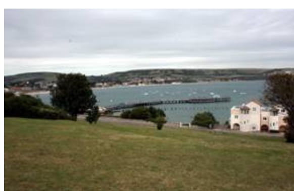
Figure 77: View of pier from Peveril Point.
