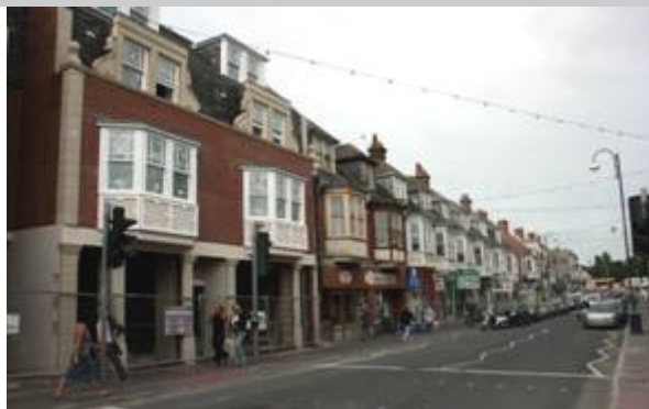
Figure 59: Edwardian shops and accommodation in Station Road.
