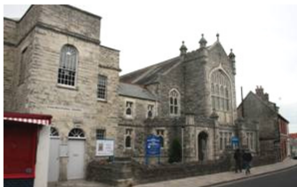
Figure 52: Swanage Congregational Church.
