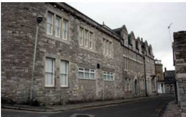
Figure 22: Swanage Water Works, Marshall Row.
