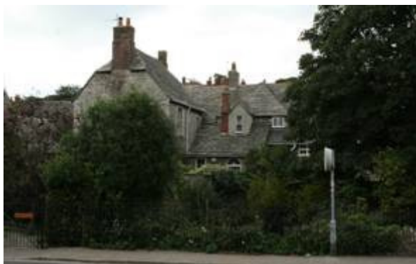
Figure 9: The Old Rectory (Swanwic House).
