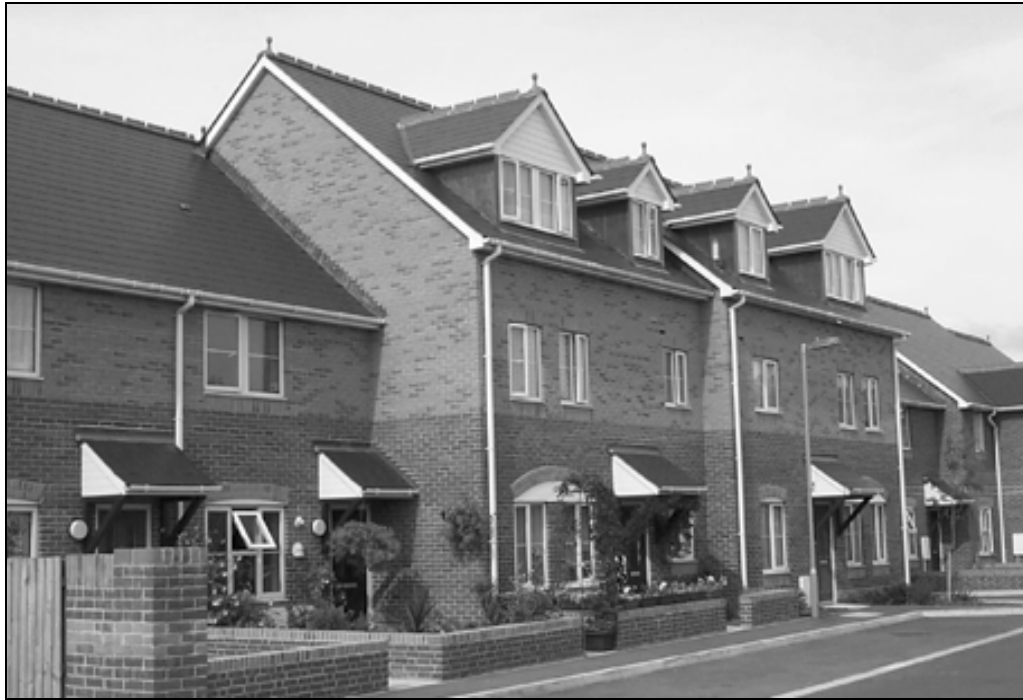
Affordable housing development at Arthur Road
