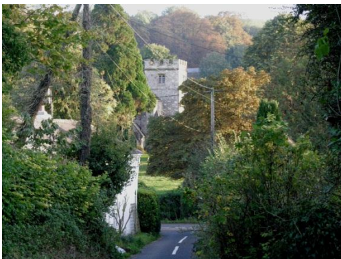
St Andrews Church Houghton
