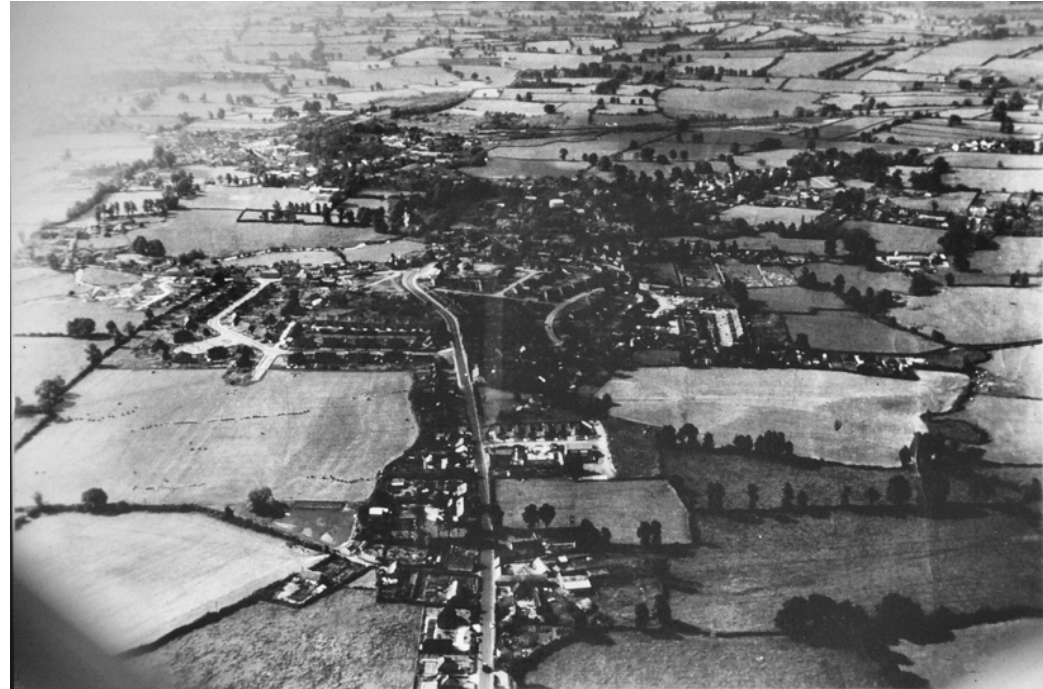
View over Peacemarsh approaching from the north and looking southward. (Arrow 1)
