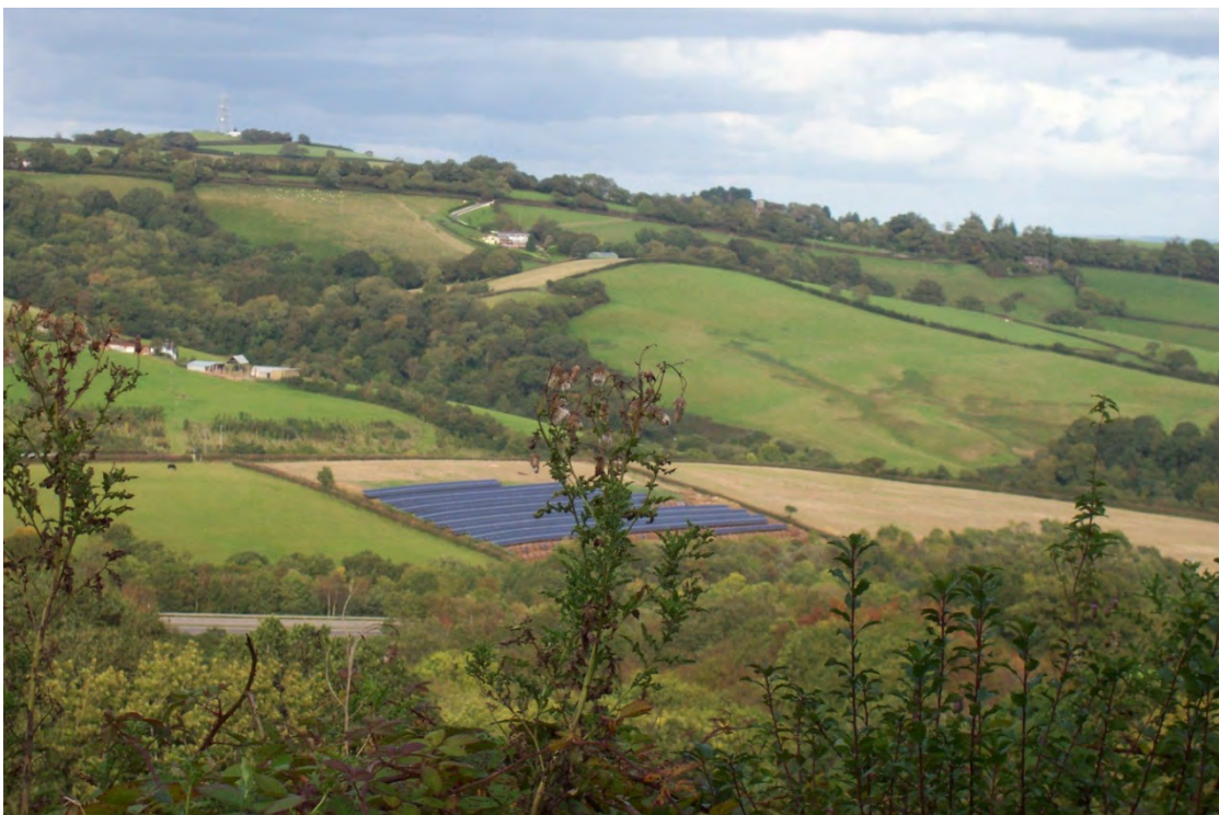
Figure 4: 1.25 hectare solar PV development at Five Mile Hill near Pathfinder Village, Cornwall
