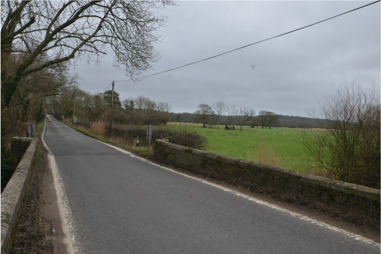
Plate 24: View of Hurst (South) Bridge
