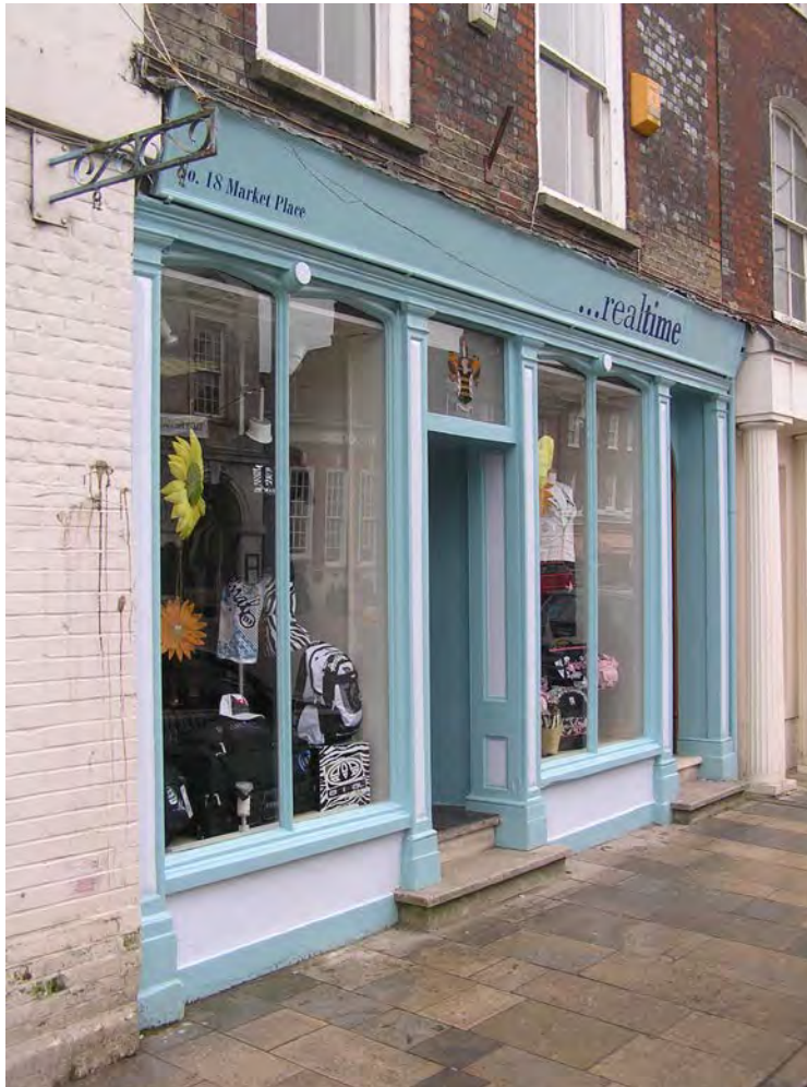
A good traditional 19th century timber shopfront in Blandford Forum
