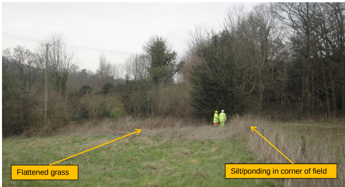
Figure 8: Fields above landslip – viewing West
