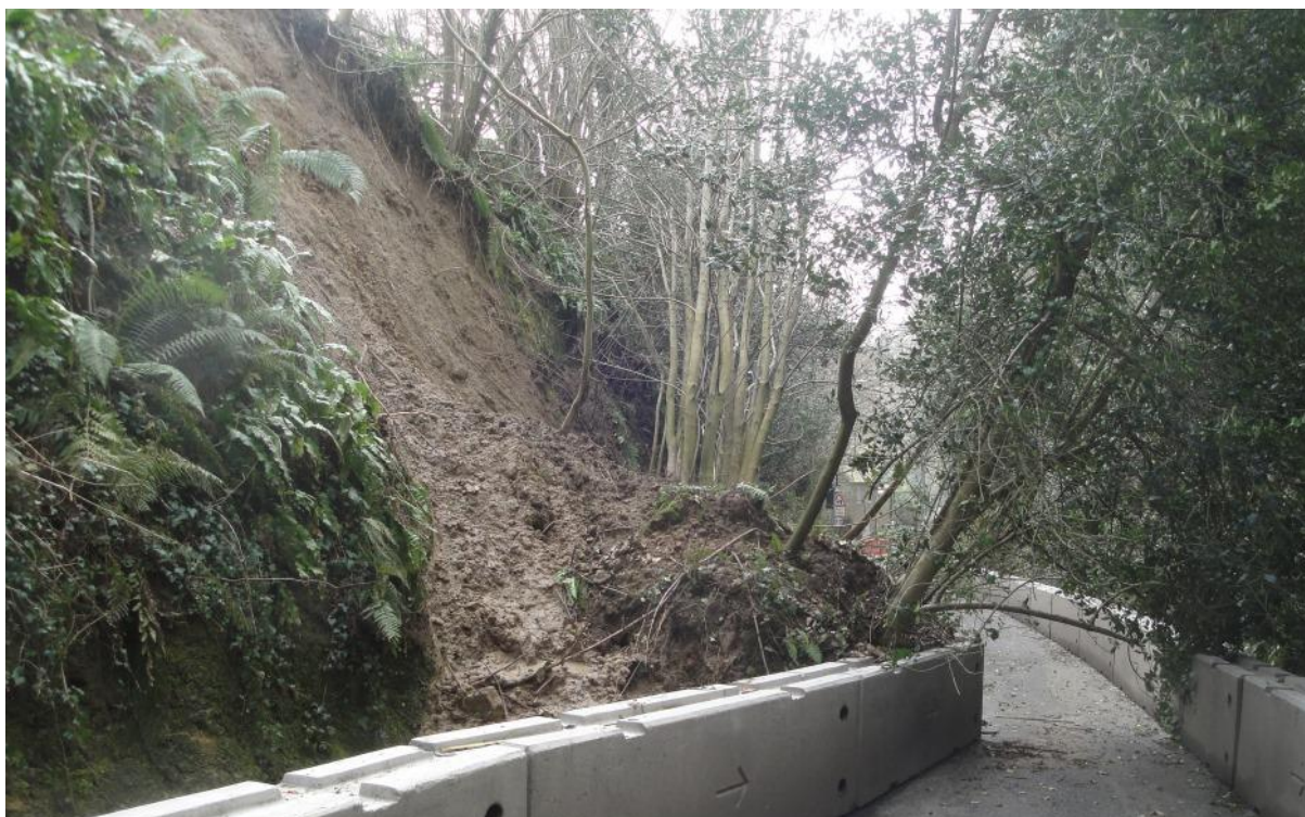
Figure 1: Landslip – viewing South
