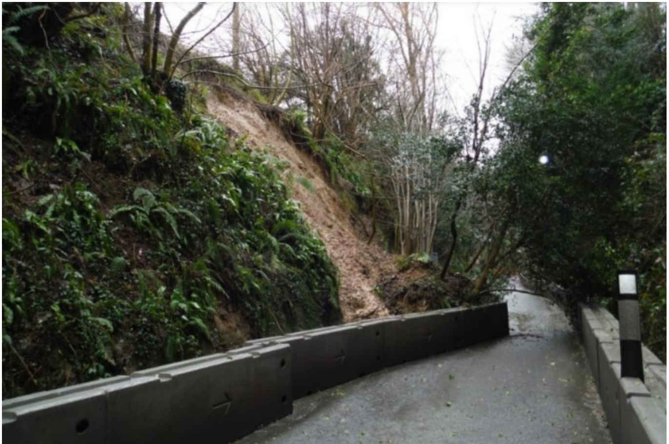
Figure 3-1 2016 slope failure
