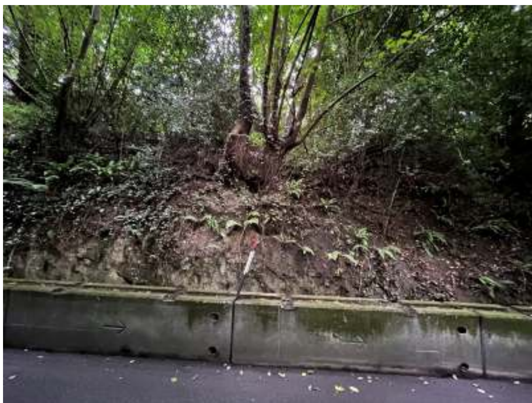
Figure 10 Eastern bank with some evidence of back scar formation.
