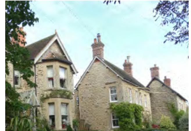
Top: Distinctive materials such as Marnhull Stone, and vernacular detailing such as the exposed roof purlins
