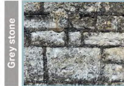
Rough course stone that has a darker hue than the Marnhull stone
