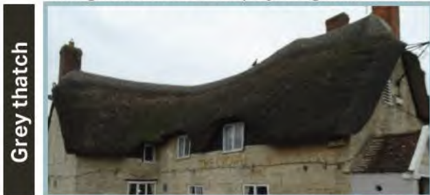
Crossed gable thatch roof with eyebrow dormers and a gable simple clay tile porch roof.
