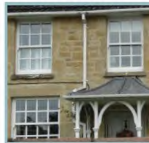
Sash window with wooden frames and glazing bars.
