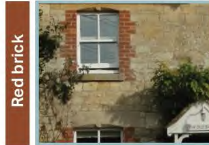
Semi-course Marnhull stone with limestone cill and brick dressing.
