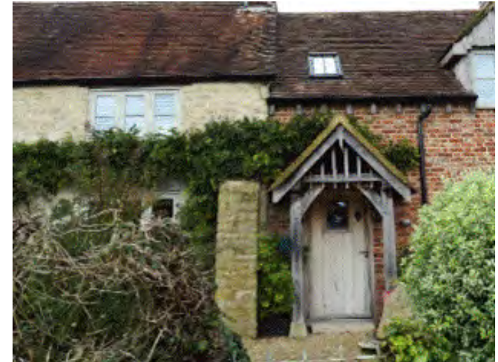
Example of how brick, wood and stone complement each other in a single building and reduces its perceived bulk
