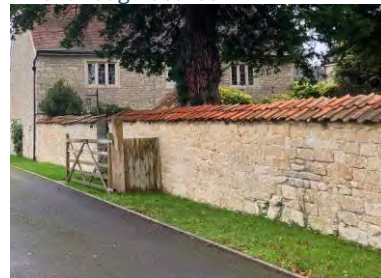
(2) red barrel tile-capped stone, of a rough course
