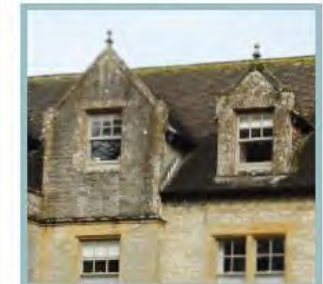
Gable wall dormer (left) and roof dormer (right) aligned with lower windows.
