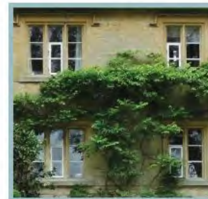
Casement window with chamfered stone mullions.
