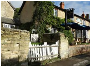
(1) round mortar-capped stone with low brick wall
