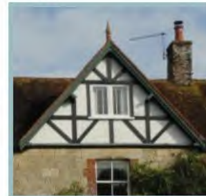
Exposed timber gable structure painted black and exposed purlins.
