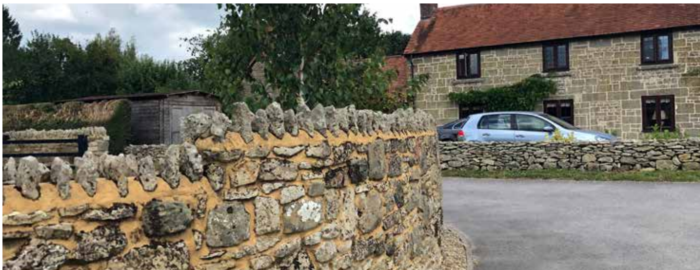
Examples of sandstone boundary walls: pebble with mortar and vertical coping (foreground) and drystone (background).
