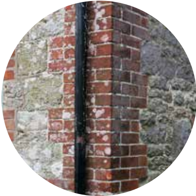
Sandstone infill with red brick trim
