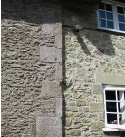
Different types of sandstone treatments and cuts: ashlar quoins and lintels with rubble infill.
