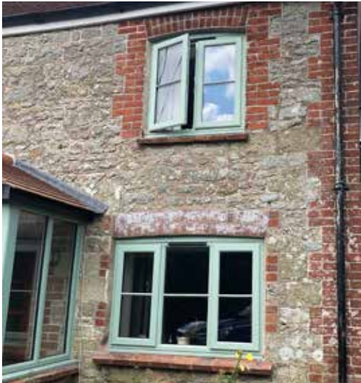
House with red brick quoins and window lintels and sandstone rubble infill.
