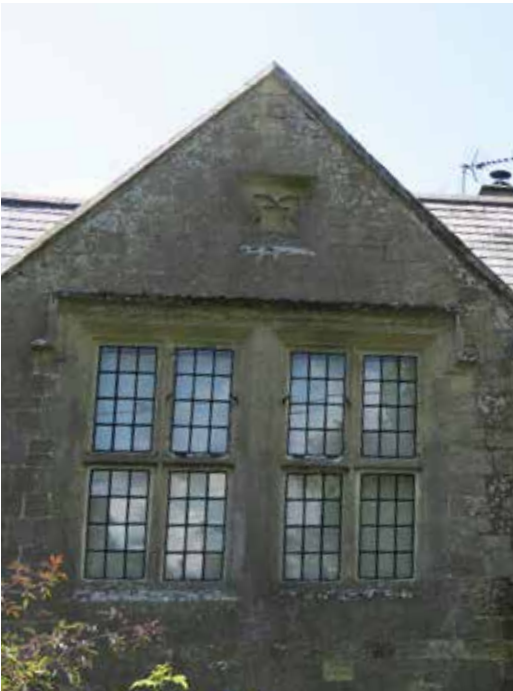
Ashlar parapet gable with mullioned and transomed stone window with hood mould.
