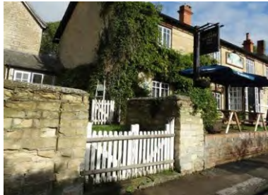
(1) round mortar-capped stone with low brick wall
