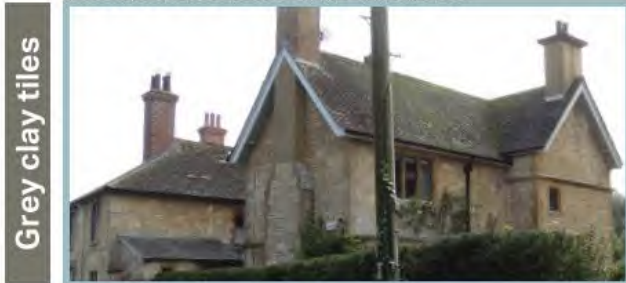
Crossed gable-roof (foreground) and hipped roof (background) with a lower projecting skillion roof.
