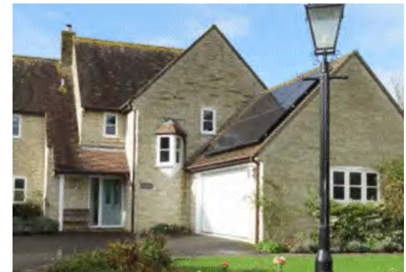
Solar panels placed discreetly in relation to the building and street
