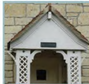
Detailed wooden gable front porch with tile roof.
