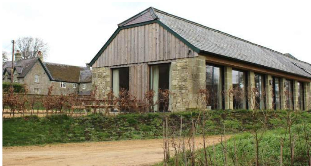
Figure 37 Example of a successful historic building conversion
