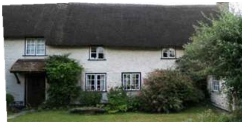
Figure 53 The Glyn Arms today (Grade II listed residential, AECOM)
