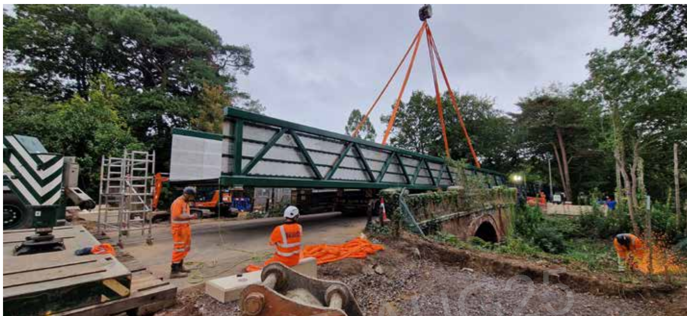
New active travel bridge being installed next to the road bridge over the railway line in Glenferness Avenue Bournemouth as part of Transforming Travel corridor.
