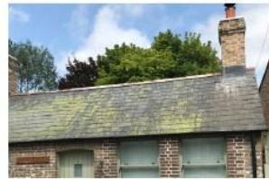
Gabled roof with grey slate tiles
