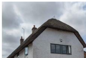
Half hipped thatched roof
