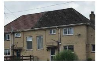
Hipped roof with clay tiles
