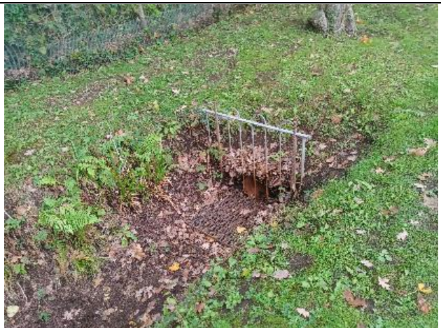
Photograph 6. Culvert beneath the access to the site.
