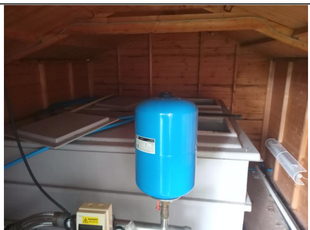
Photograph 12. Internal area of the treatment shed in the north of the site.
