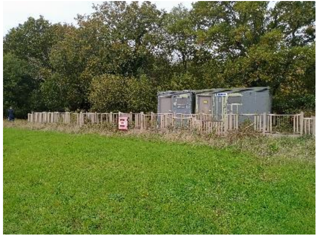
Photograph 2. Derelict facilities building in the northwest of the Site.
