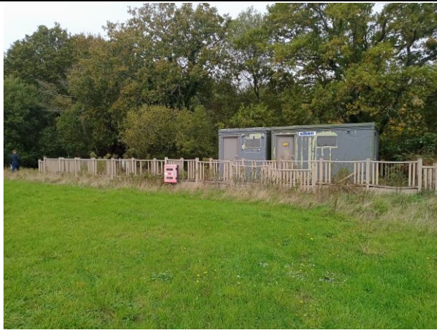
Photograph 7. Derelict toilet block in the northwest of the site.
