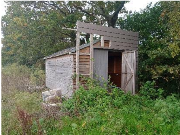
Photograph 1. Shed housing water supply tank in the central north of the Site (previously a facilities building).
