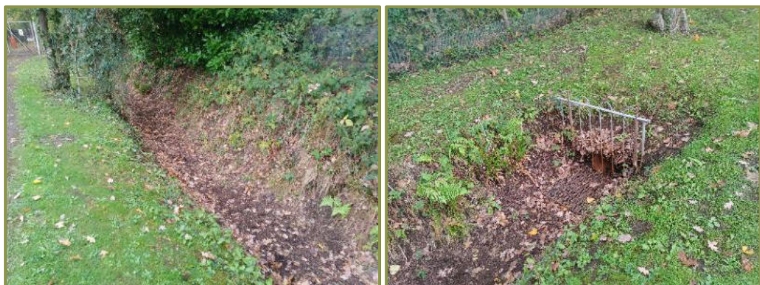
Left: Watercourse 1. Right: Culvert.
