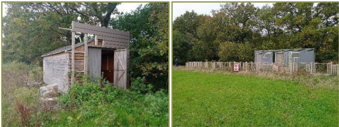
Left: Shed housing water supply tank in the central north of the Site (previously a facilities building). Right: Derelict facilities building in the northwest of the Site.
