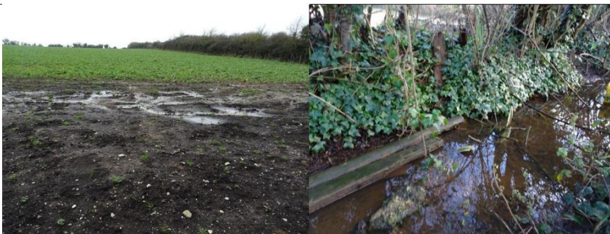
Looking towards crest of square field
