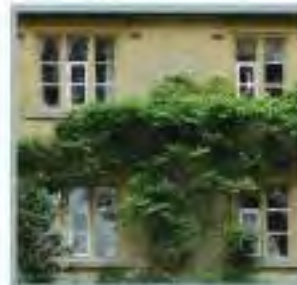
Casement window with chamfered stone mullions.
