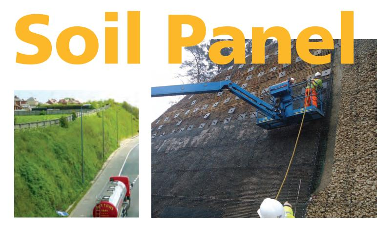
Soil Panel was designed and patented by Phi Group to be used specifically in conjunction with Soil Nails where the creation of extra space requires existing embankments to be cut back forming steep sloping faces. Whilst soil nailing provides the principle structural support to the cutting, Soil Panel steel cages provide a flexible facing which can provide structural support as well as facilitating an excellent finish
