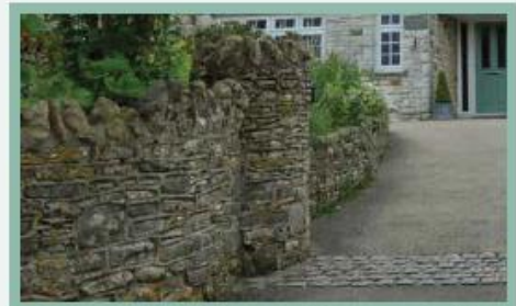
Stone wall with lime mortar topped with larger 'cock and hen' cap stones.
