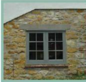
Painted timber casement window with stone lintel
