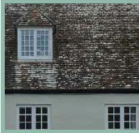
Hipped roof dormer aligned with lower level windows
