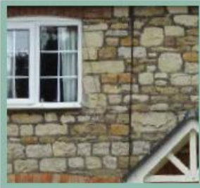
Coursed rubble-stone wall
