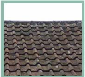
Double Roman interlocking roof tiles
