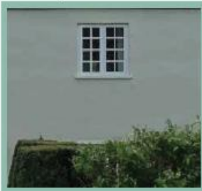
Light coloured render over rubble-stone walls
