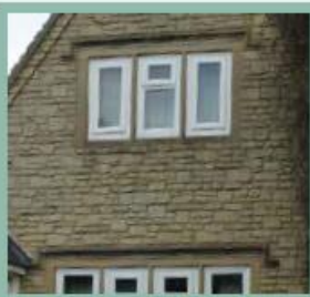
Stone hood moulds consistent over all windows
