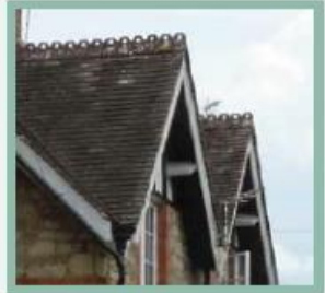
Simple handmade clay roof tiles topped with ridge tiles
