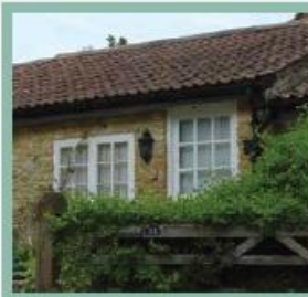
Timber casement windows flush with the outer wall
