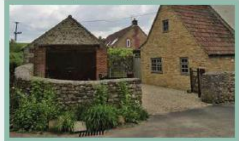
Rounded mortar capped wall enclosing the dwellings whole curtilage area.
