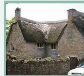
U-plan thatched roof with gable ends
