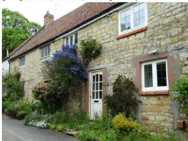
Figure 23: 1 & 2 East Farm Cottages: Two attached cottages directly fronting North Street with varying fenestration detailing and a continuous Roman interlocking roof tile distinct from other cottage vernaculars from the 17 th C within the area.
