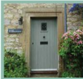
Plank door set within a stone dressing
