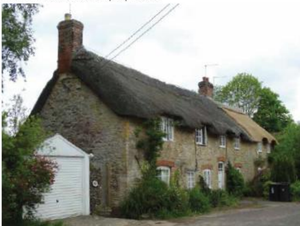
Figure 29: Greenfields, Bankside and Wild Thyme Cottages: a row of three Grade II listed terraced buildings featuring coursed rubble-stone walls, thatch roof with gable ends, wooden casement windows and cambered brick arched lintels.
