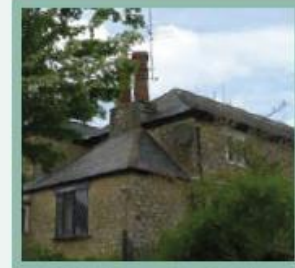
Slate hipped roof with integrated side range
