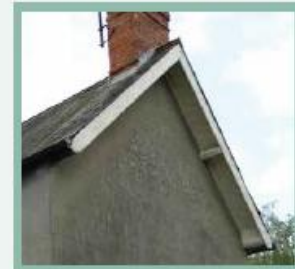
Overhang verge with a soffit of diagonal timber boarding
