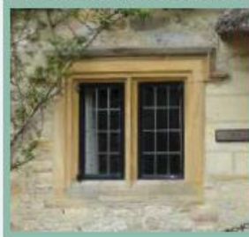
Iron casement window with chamfered stone mullions
