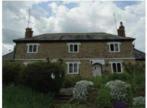
Figure 26: 3 & 4 Westbury: Grade II listed semi-detached cottages featuring a coursed local lias stone facade with ashlar dressings, windows with metal casements and hood moulds, hipped slate roof and attached side ranges on each end.
