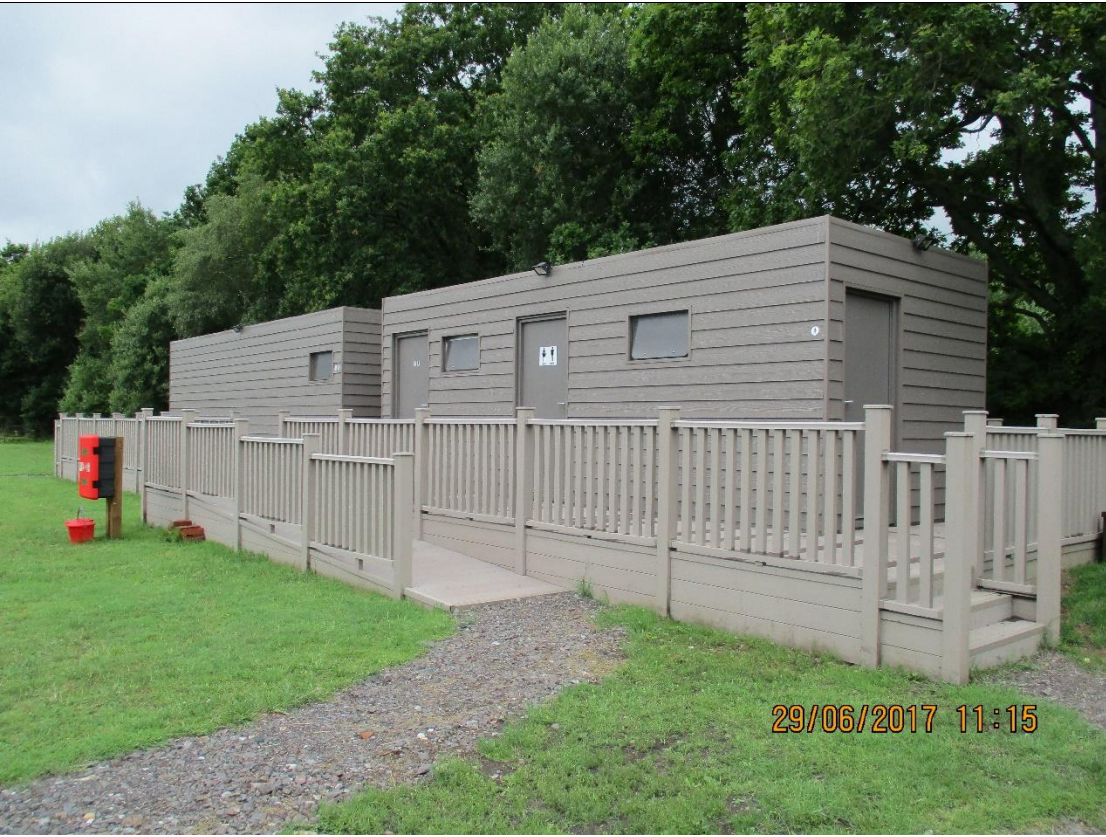
29.06.2017 Toilet Block and fire point
