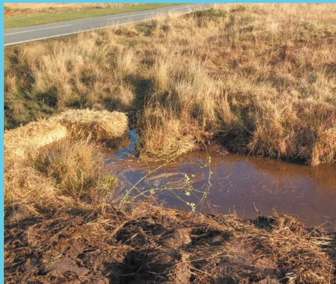
Straw bales acting to prevent siltation downstream © Mair Rees
