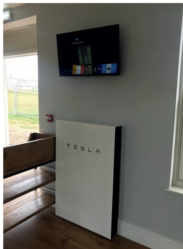
Battery storage gives greater control over how and when you use the energy you generate, allowing you to replace the electricity you buy from the grid with the free electricity your panels are generating. It also provides a back-up in the case of power cuts and ensures the café's fridges and freezers keep running.
