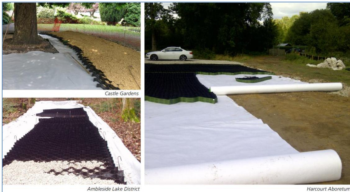
**Figure 3:** example cellular confinement system.
