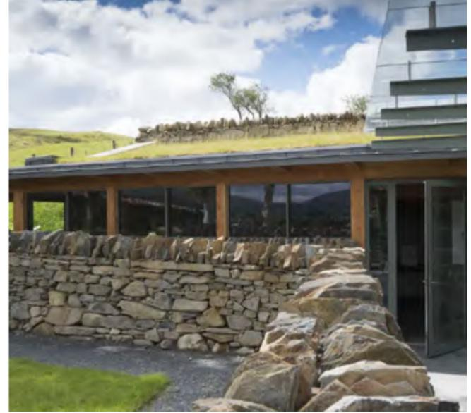
A natural muted material palette of the spa on the southern boundary is linked to the architectural character of the surrounding rural area with Purbeck stone forming the walls and timber brise soleil to act as solar shading. This specification would readily be available within the local area. The roof will be covered in local heather and grasses to match the existing character of the Studland landscape.
