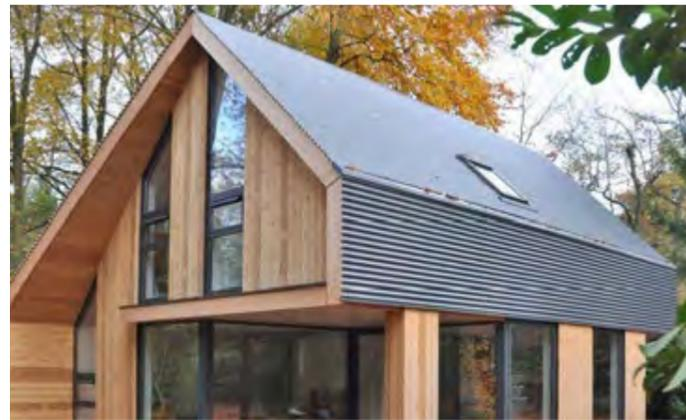
Design precedent - timber cladding and metal roof
