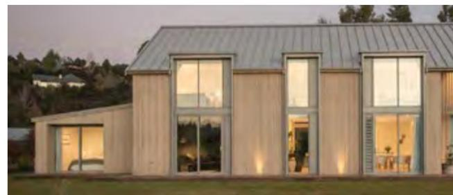
Contemporary dormer windows punctuate a standing steam roof adding visual interest and providing greater daylight internally
