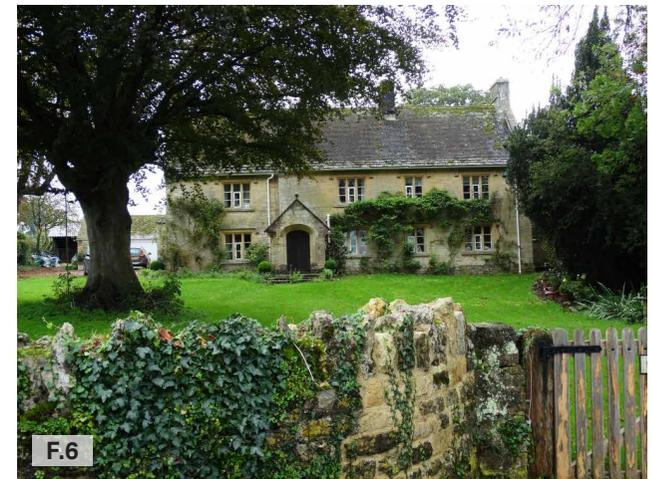
Figure 06: Example of a coursed square rubble facade.
