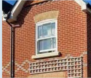
Sash window including stone sill and feature window arches
