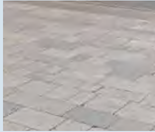
Stone paviours (Market Place)
