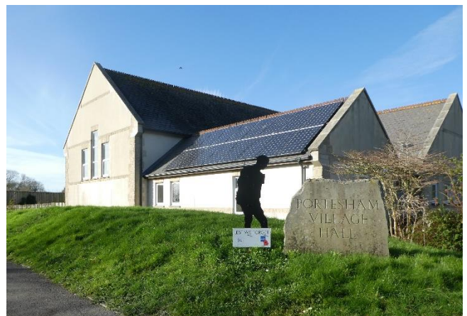
Figure 17: Portesham Village Hall
