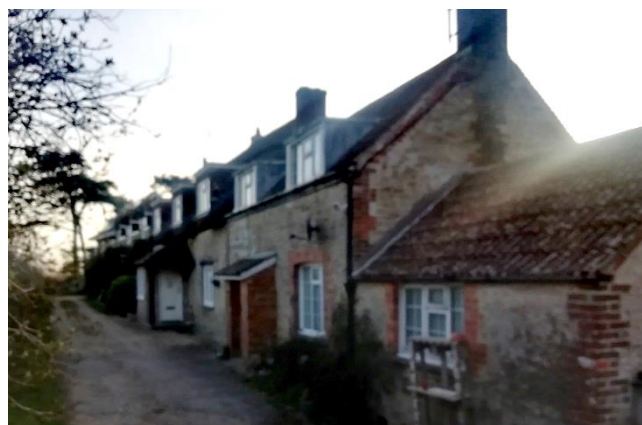
Figure 3: Cottages in Butter Street, Fleet
