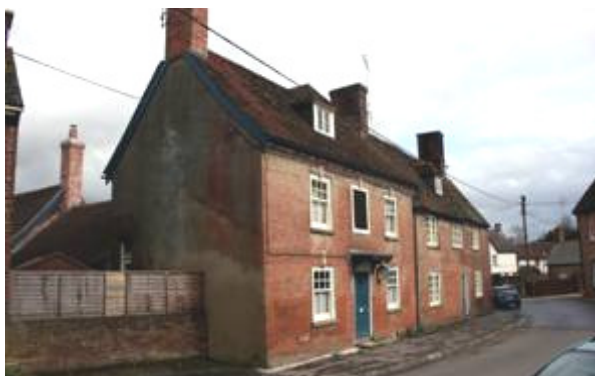
Figure 50: Nos 2 and 4 Salisbury Street .
