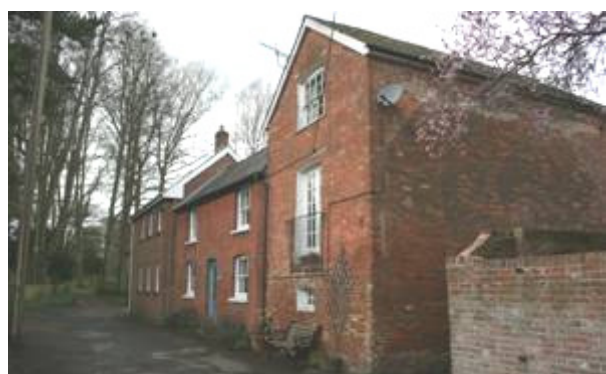
Figure 47: Old Granary, Swan Street.
