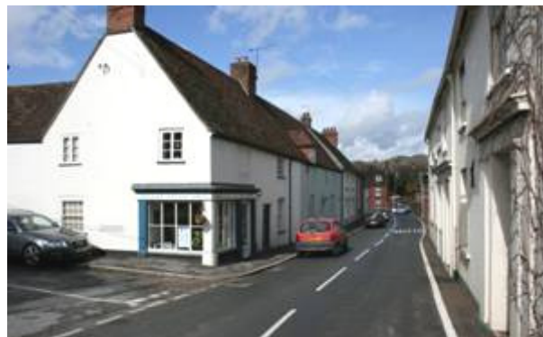
Figure 42: View north along Wimborne Street .
