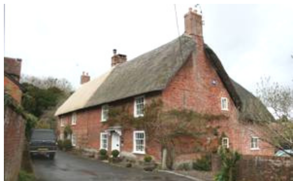
Figure 46: Nos 1 and 2 Church Street.
