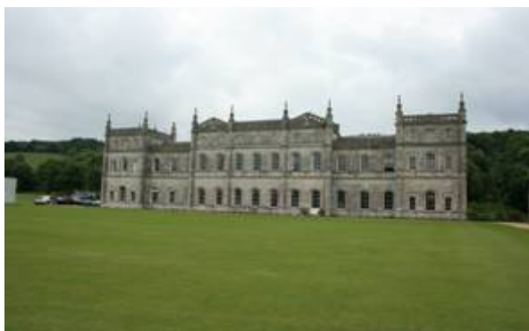
Figure 27: Milton Abbey House, west front.
