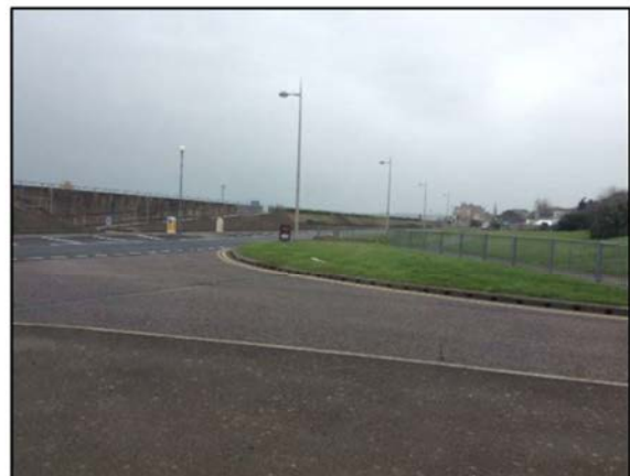
Highway access and sea wall
