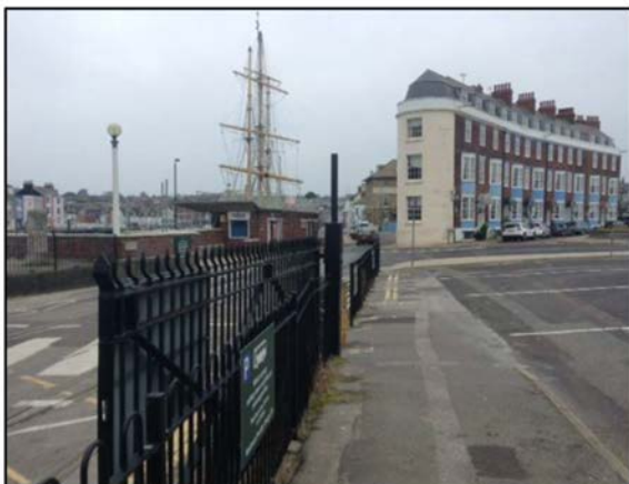
Devonshire Buildings Gateway to site
