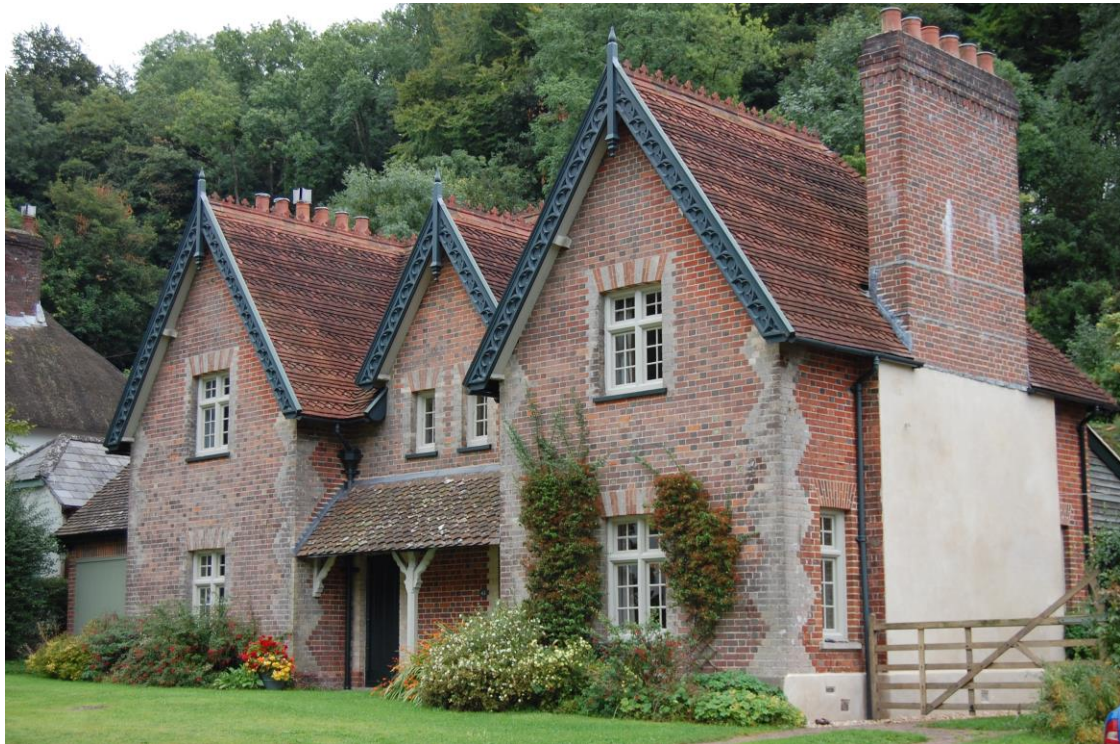
The 19 th Century replacement Cottages
