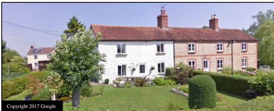
Fig 41. Purns Mill Cottage and Riverside Cottage
