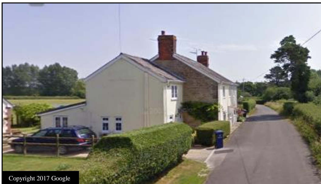
Fig. 31 Purns Mill Cottages
