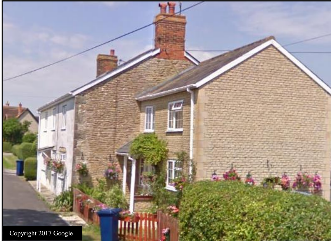
Fig. 30 Purns Mill Cottages
