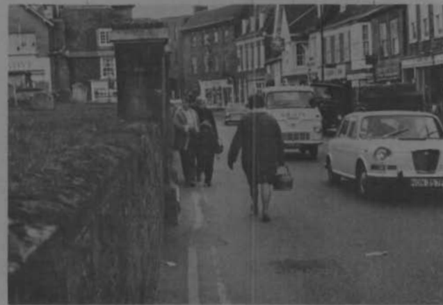
Dangerous lack of pavement.
