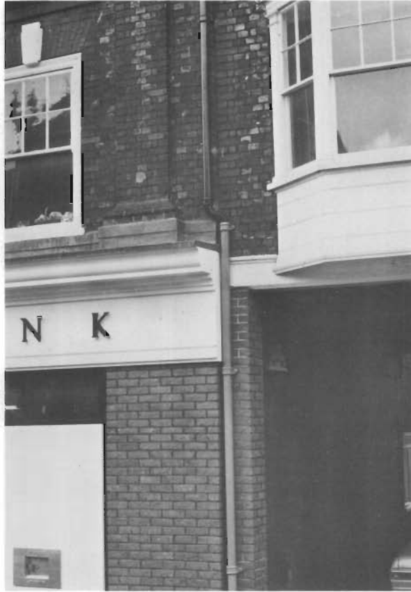
Old and new brickwork.
