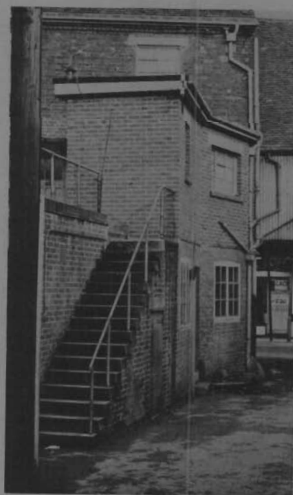
Private access to upper floor.
