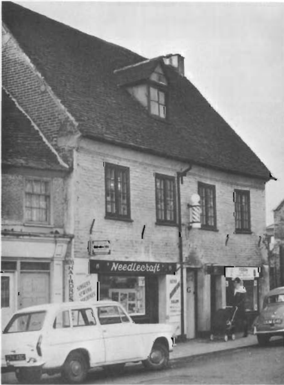
Nos. 15 and 17 East Street.
