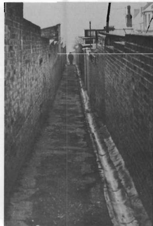
Bury the gutters and pave.
