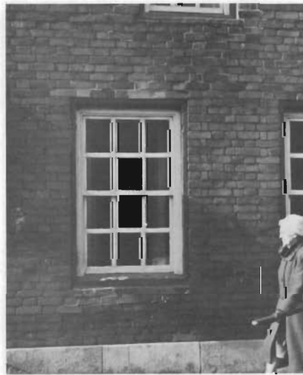
Thick glazing bars of early sash window and mathematical tiles.
