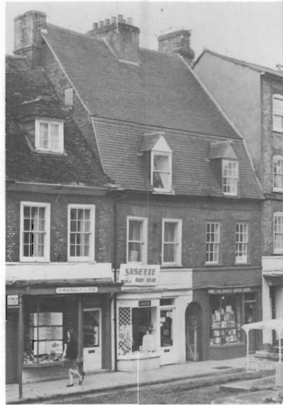
Note lost glazing bars above "SUSETTE".
