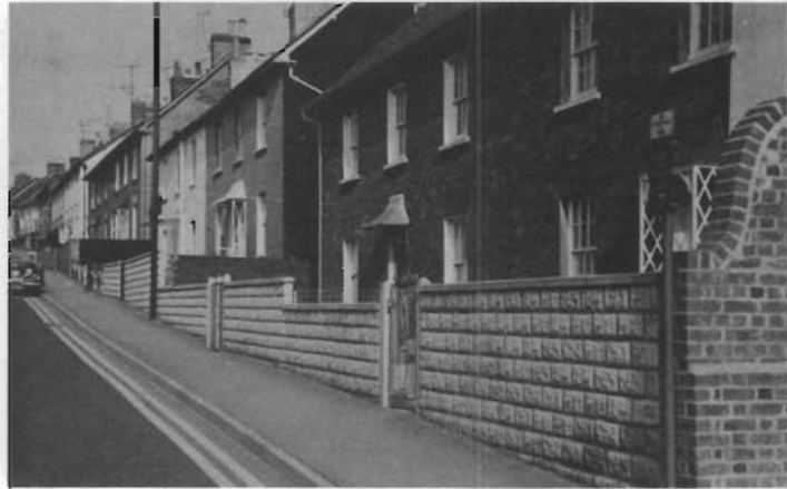
Rusticated artificial stone walling should be forbidden in the Conservation Area.
