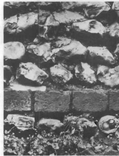
A badly pointed brick and flint wall - as it should be.
