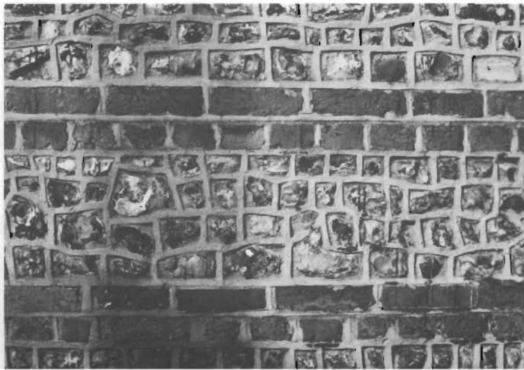
A badly pointed brick and flint wall - as it should be.
