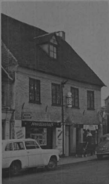
Nos. 15 and 17 East Street.
