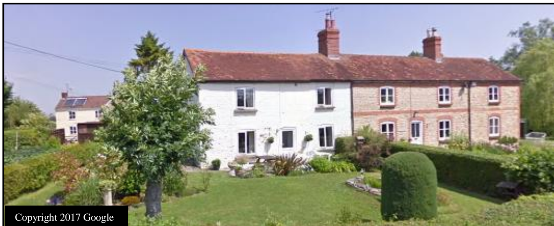
Fig 41. Purns Mill Cottage and Riverside Cottage
