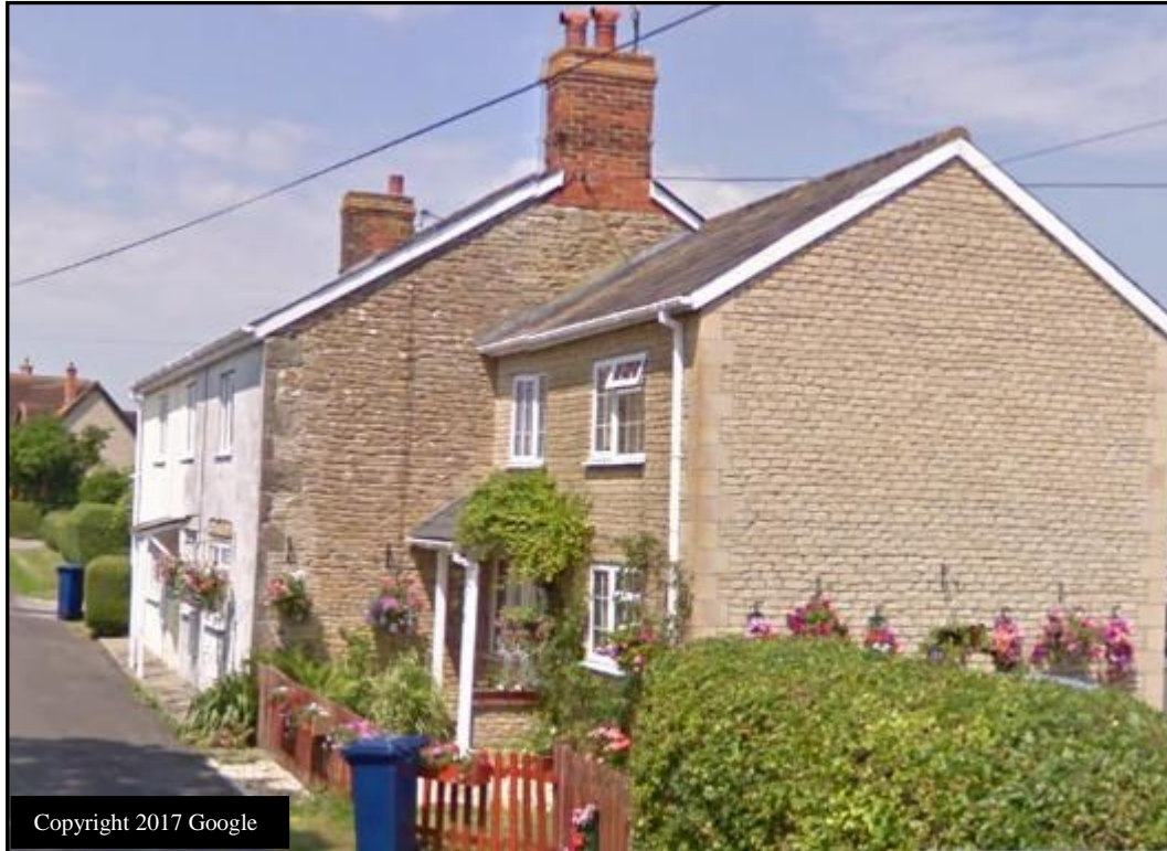
Fig. 30 Purns Mill Cottages
