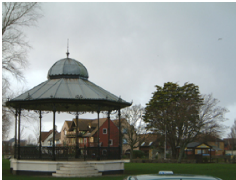
The Bandstand on the Quomps
