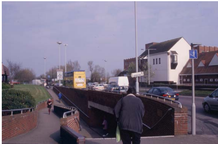
Underpass to Fountain Way
