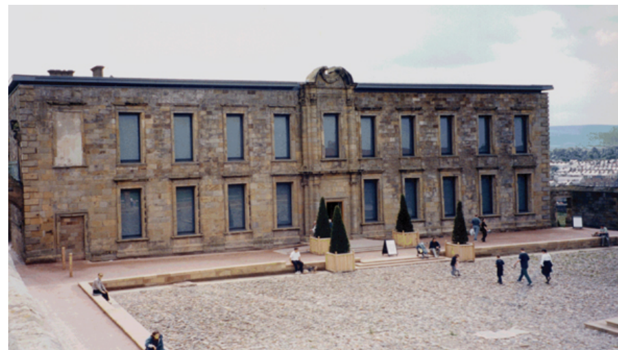
Cholmley House Visitor Centre, Whitby
