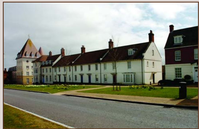
Affordable housing, Poundbury Phase I, Mansell Square
