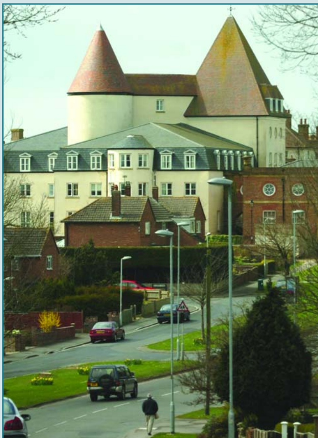
Fleur de Lis Phase I (looking west)
