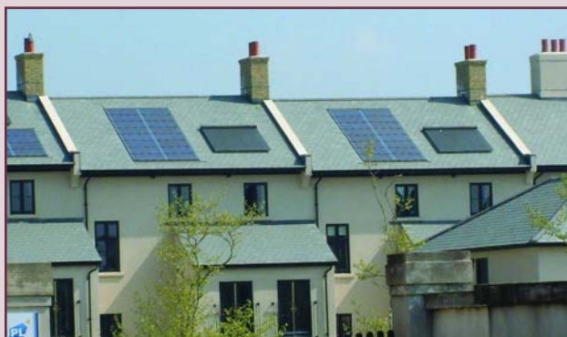
Solar panels and photovoltaic cells on south facing roof slopes
