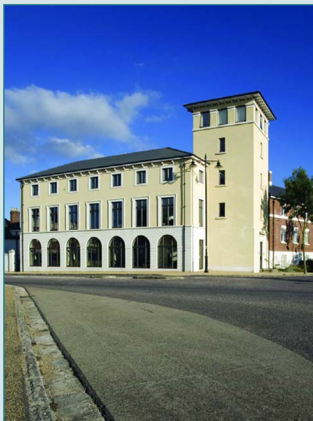
Armitage House, Victor Jackson Square. A smaller landmark building.
